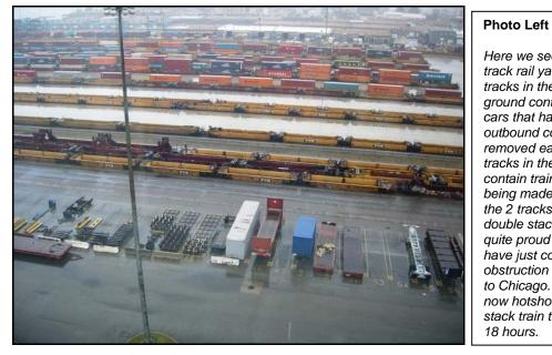
Here we see the 12 track rail yard. The tracks in the foreground contain the cars that had their outbound containers removed earlier. The tracks in the distance contain trains that are being made up. Notice the 2 tracks that contain double stack cars. NS is quite proud that they have just completed an obstruction free corridor to Chicago. They can now hotshot a double stack train to Chicago in 18 hours.
