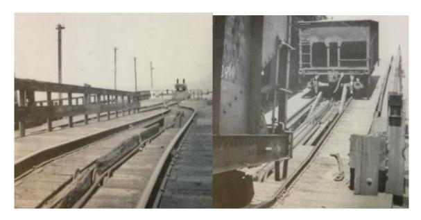
At the apex of the incline the cars rolled through spring switches to a sharp incline which "kicked" them back down the upper level grade of 1.5 inch per 12 feet, to the coal pockets, where a brakeman, riding the car would "spot" it. After unloading the car would be allowed to roll unattended to the yard.
