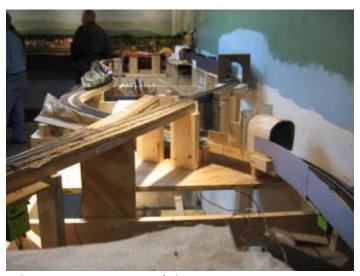
Spline construction on Jim's layout. (Photo by Dennis Blank)
