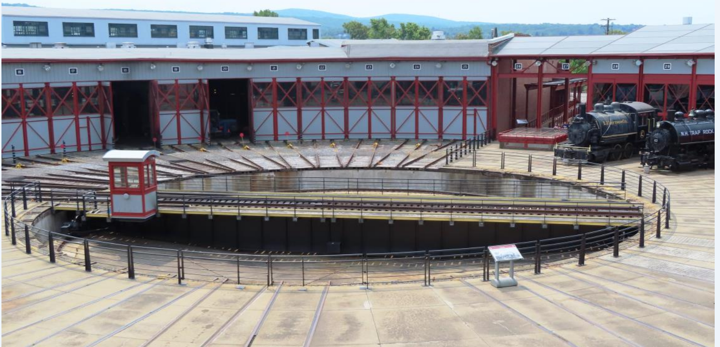
turntable and roundhouse at Steamtown National Historic Site, Scranton, PA
