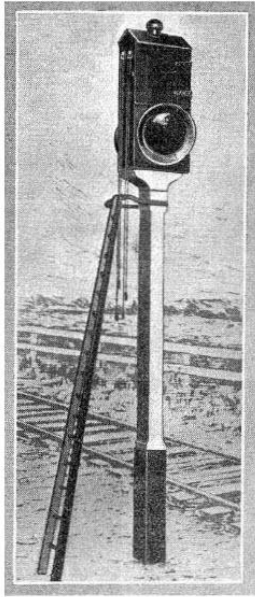
Banner box signal installed in 1863 between Philadelphia, Pa., and Trenton, N. J. First type of manual block signal put in service in the United States
